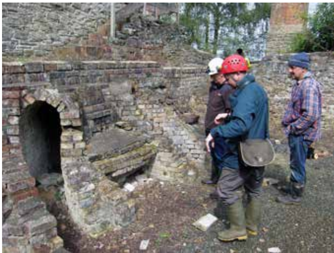
The compressor boiler house. Photo Tim Wellburn
